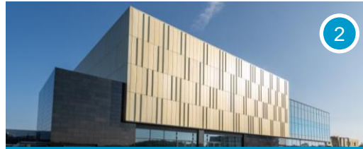
Modern commercial & retail: The Springs
